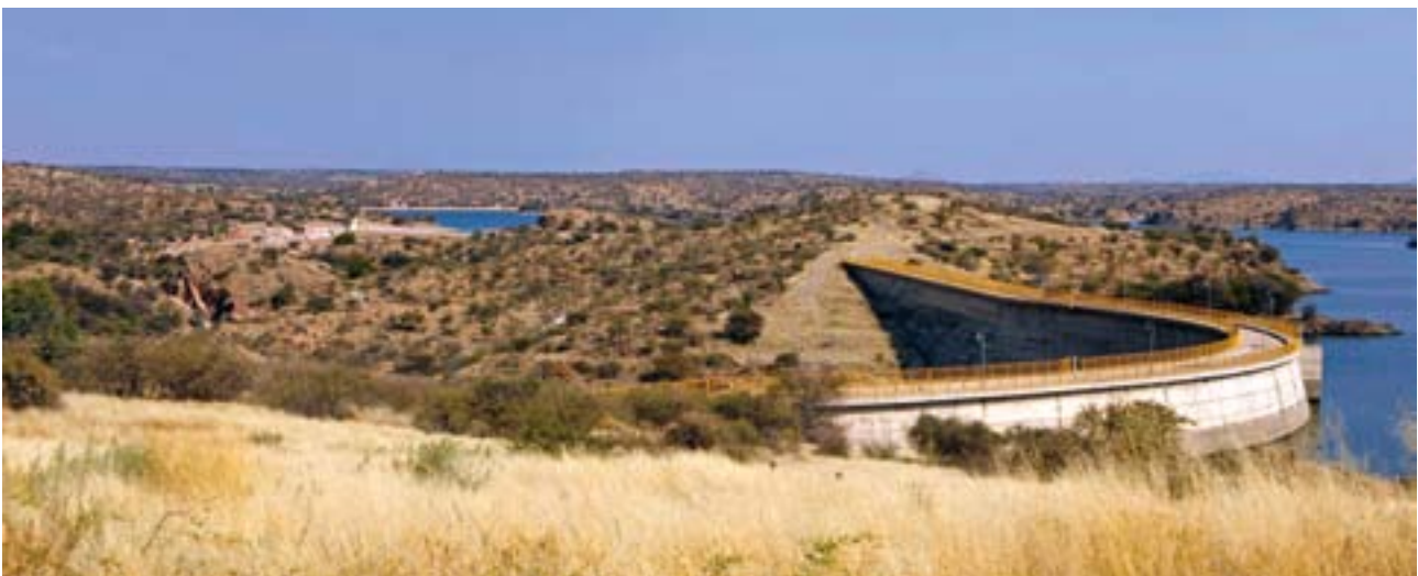
Oanob Dam is a double-curvature arch dam on the Oanob River, Namibia, that supplies the town of Rehoboth via a four-kilometre pipeline.
