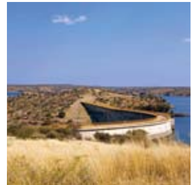
Oanob Dam is a double-curvature arch dam on the Oanob River, Namibia, which supplies the town of Rehoboth via a four-kilometre pipeline.
