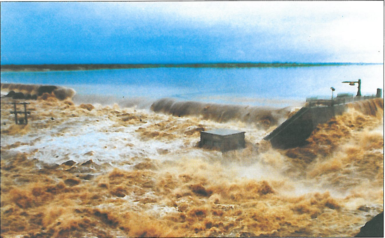
Spitskop Dam, breached due to overtopping by the February 1988 flood, with side-channel spillway on the right (Harts River)
