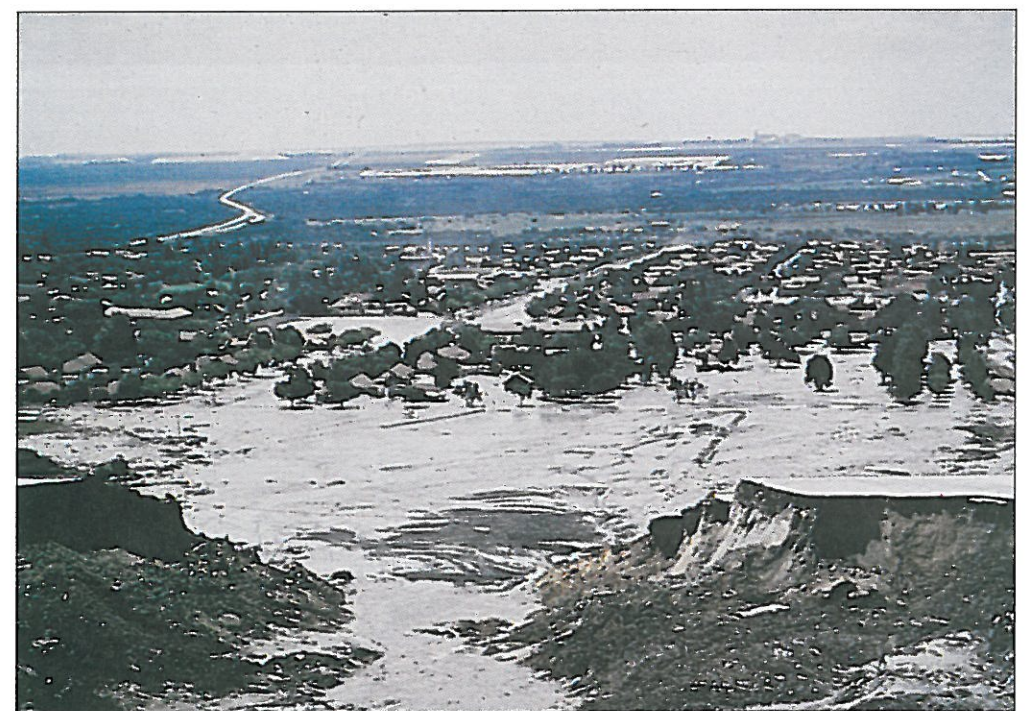
Harmony Gold Mine tailings dam failure (February 1994 ) and flooded town of Merriespruit, Virginia, OFS
