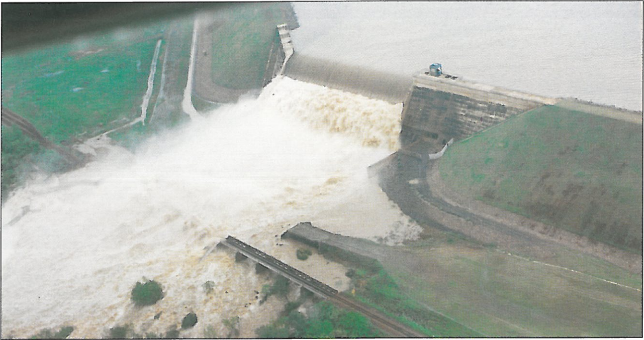
Albert Falls Dam during the September 1987 flood with the washed away railway bridge downstream of dam (Mgeni River)
