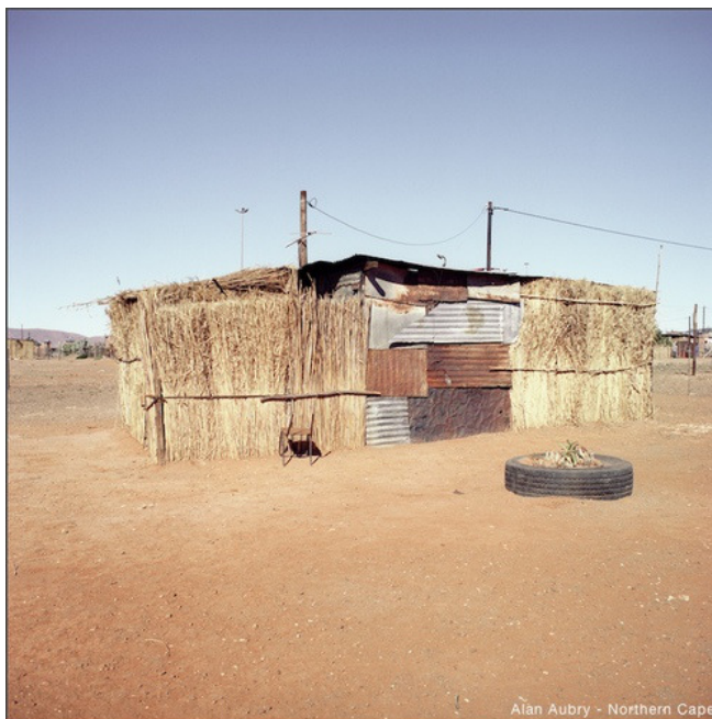
Figure 3.2: Temporary Structure made from Reeds
