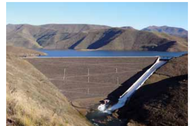
Mohale Dam, part of the Lesotho Highlands Water Project (© UNOPS/C Mor)
