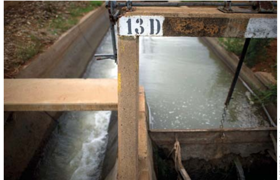
Vaalharts Storage Weir
