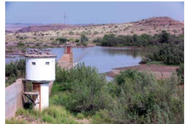
Seeheim Gauging Station on the Fish River in Namibia (© S Crerar)
