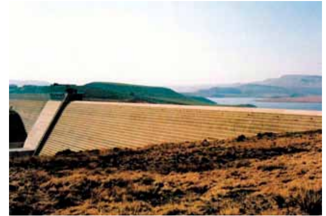
Zaihoek Dam (source: SA Dept of Water Affairs)
