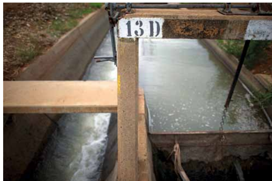
Vaalharts Storage Weir (© UNOPS/Leonie Marinovich)
