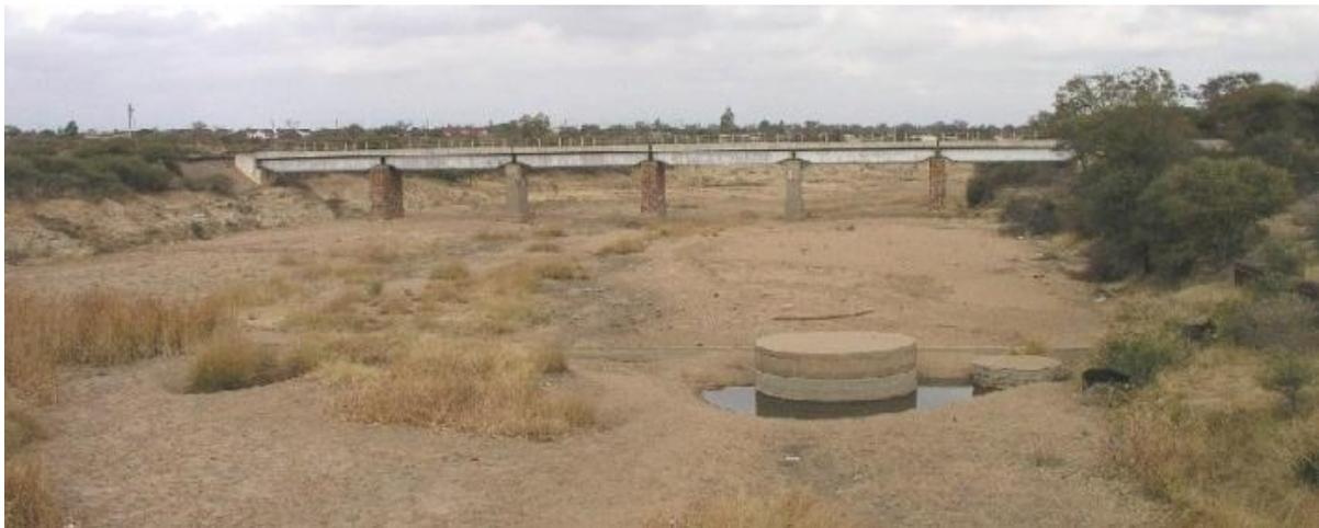
**Figure 24:** Large-diameter collector well upstream of a subsurface dam within the riverbed of a headwater tributary of the Limpopo River, Botswana<sup>vi</sup>
