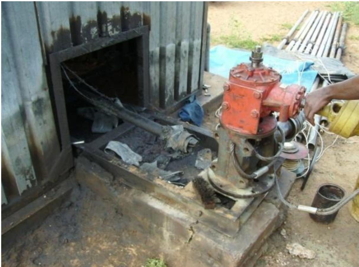
**Figure 10:** Borehole suffering from lack of O&M – diesel spillage and cracked concrete block
