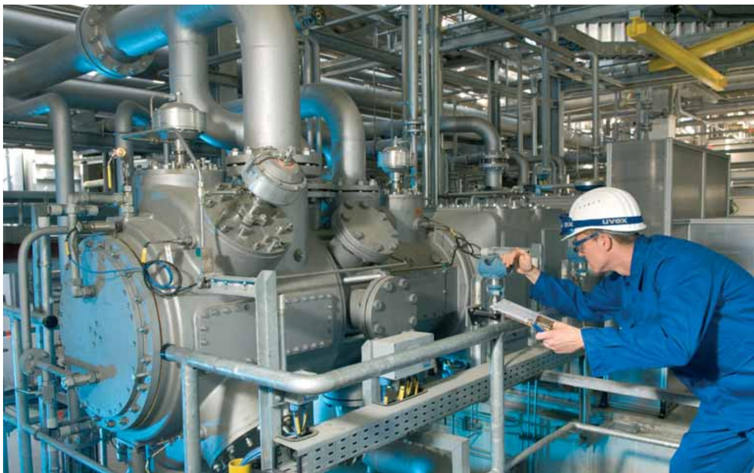
Maintenance work being conducted at the recycle gas compressor at the Sasol O&S plant in Brunsbüttel, Germany.
