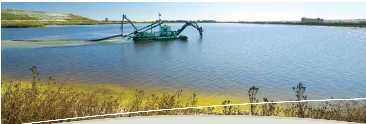
A dredger removing sediment from an evaporator dam to increase capacity for water received from Secunda plants, as well as rain water.
