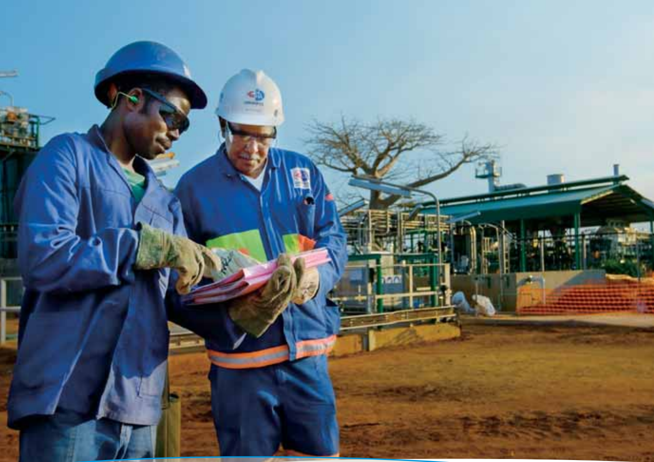
Central processing facility, Temane, Mozambique.
