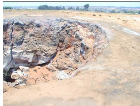
Figure 2. Surface collapse due to abandoned burning workings at T&DB.
