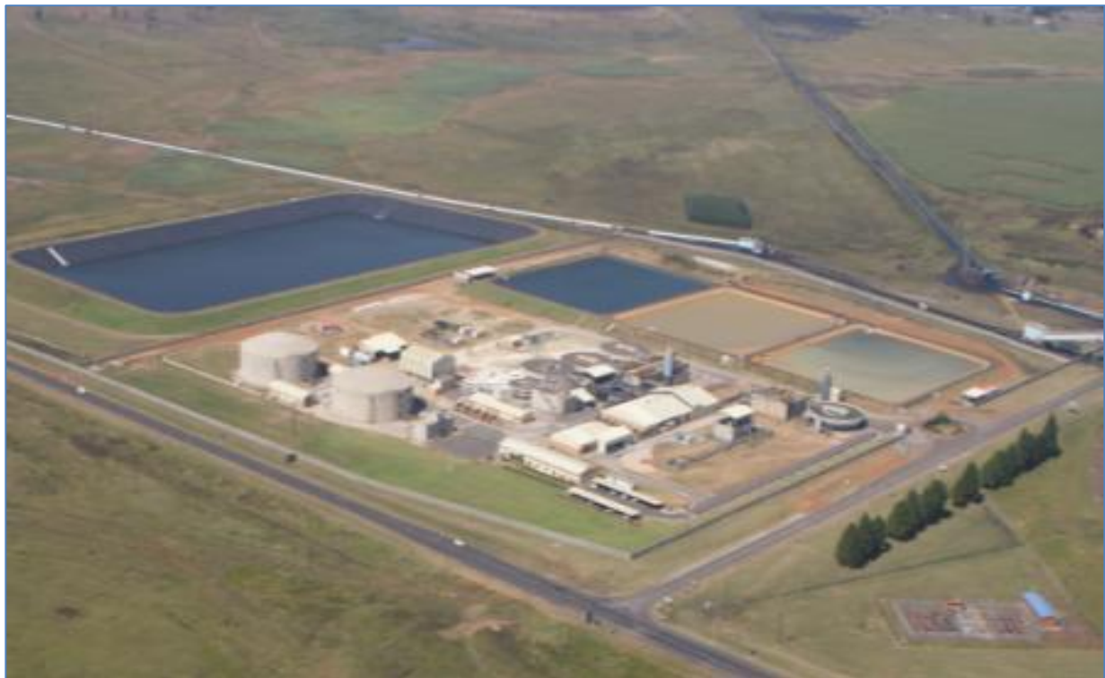
Figure 1: The existing Water Reclamation Plant associated with the eMalahleni Mine Water Reclamation Scheme
