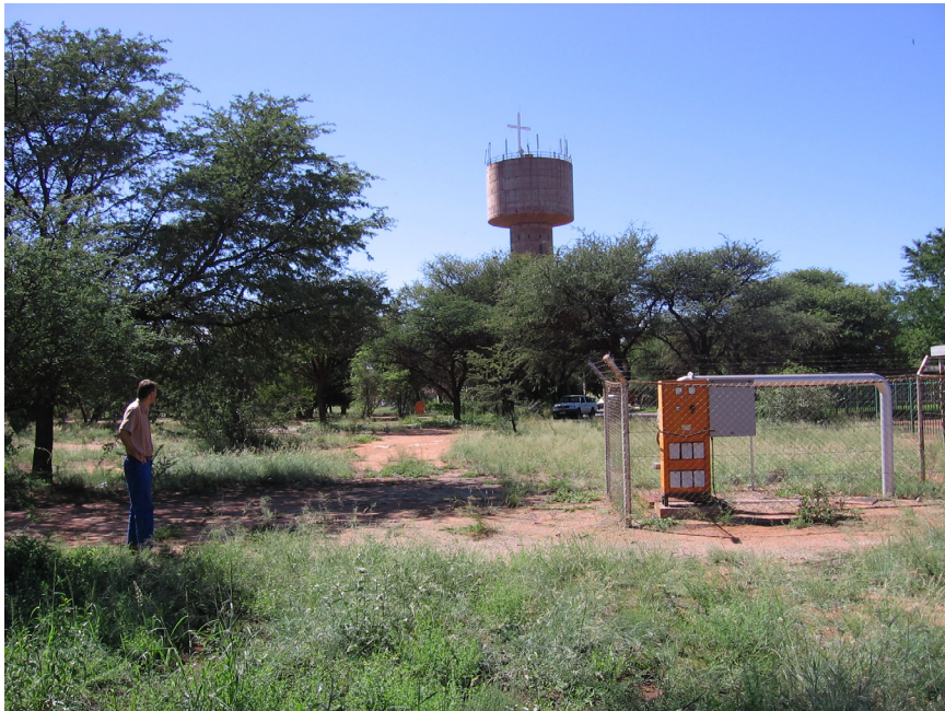
One of Kathu's production boreholes
