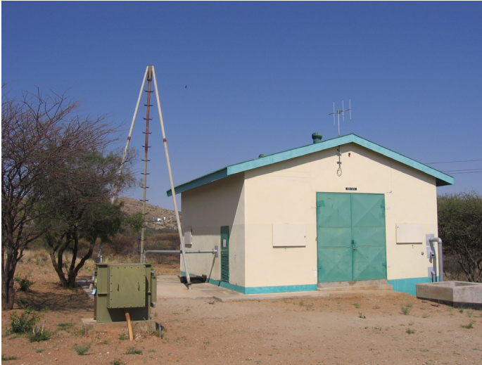
One of Windhoek's injection boreholes (below the tripod) and the water treatment building where further treatment is given through Granular Activated Carbon and chlorination
