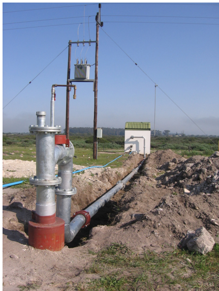
Injection borehole for pilot tests
