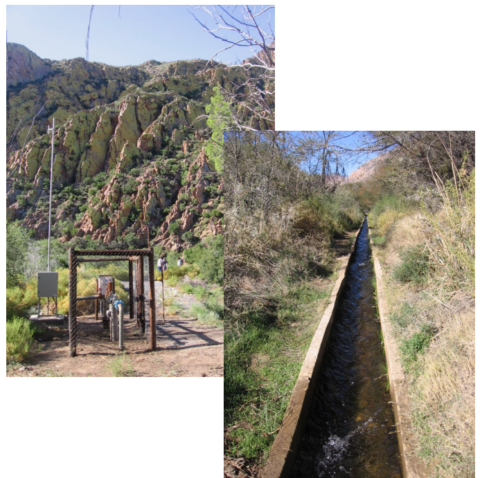
Planned Prince Albert injection borehole and source water (diverted runoff from the mountains)
