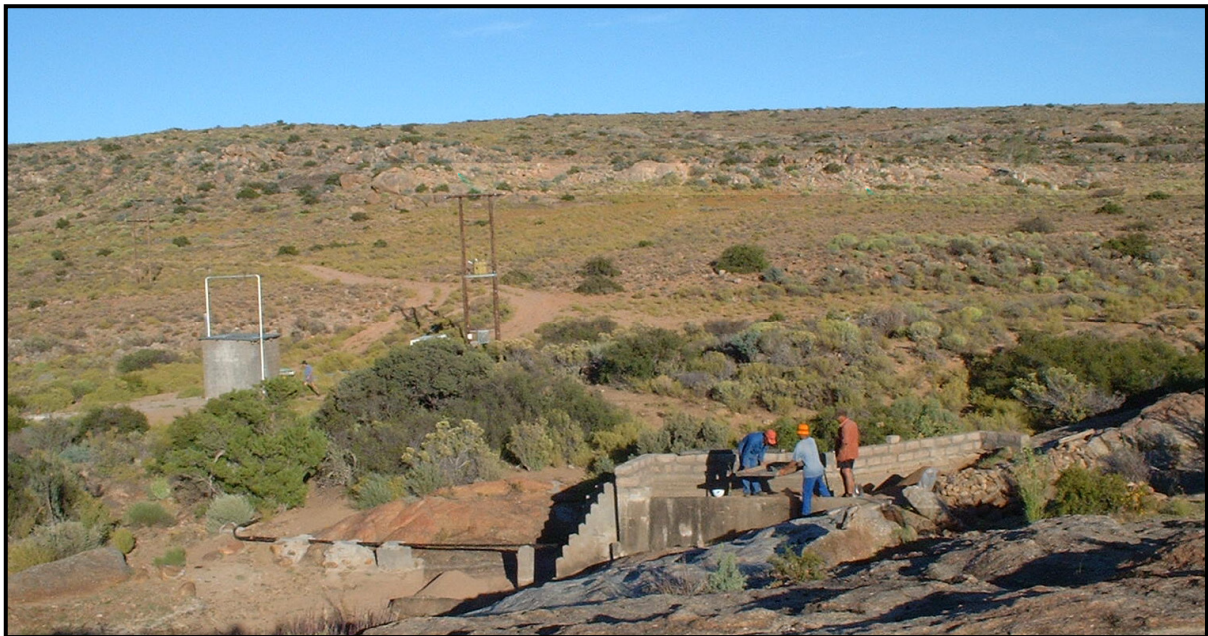
Sand filter with injection and abstraction borehole (pump house) in the background
