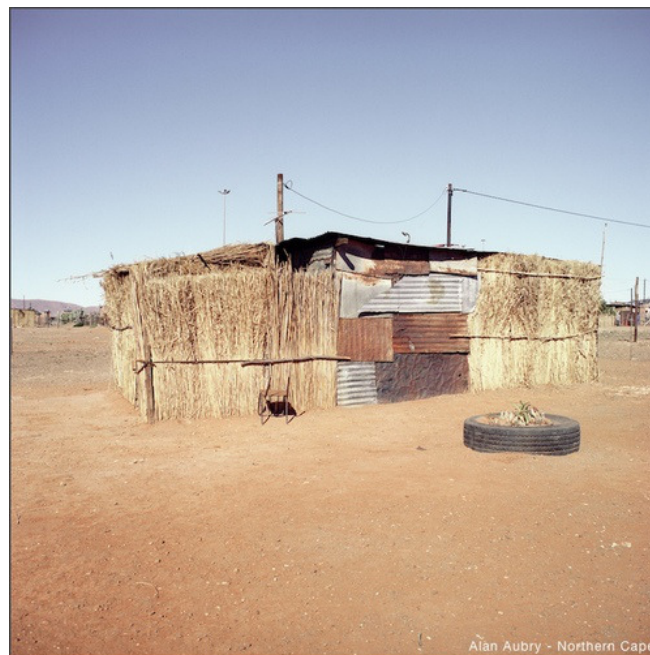
Figure 3.2: Temporary Structure made from Reeds
