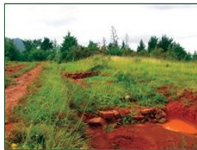
Stone dams placed in erosion dongas reduces the impacts of soil erosion. Source: Kruchem 2011 ( click to enlarge )
