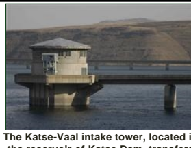
The Katse-Vaal intake tower, located in the reservoir of Katse Dam, transfers water from Katse Dam, through Muela Power Station to the Vaal River. Source: Vogel 2009 (click to enlarge)
