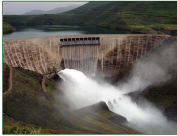
Katse Dam, the keystone of the Lesotho Highlands Water Project.
