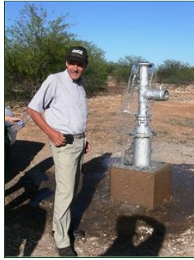
An artesian borehole in the Stampriet area of Southern Namibia. Source: Kirchner 2008 ( click to enlarge )
