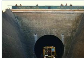
The Orange-Fish transfer tunnel. Source:DWAF South Africa 2009 (click to enlarge)
