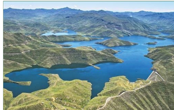
Mohale dam is a rock-fill dam constructed on the Senquyane River that comprises the major component of Lesotho Highlands Phase 1B. Source: Lesotho Highland Development Authority 2006 ( click to enlarge )
