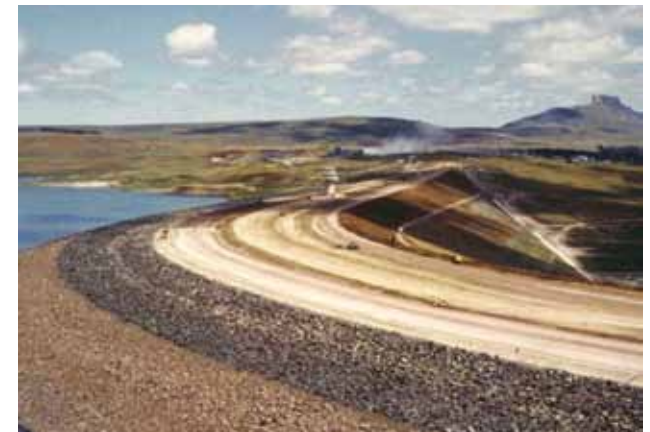
Sterkfontein Dam under construction. (Source: SA Dept of Water Affairs)
